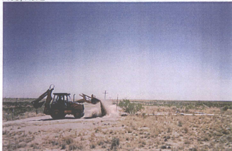
Backfilling with clean imported soil, facing east
