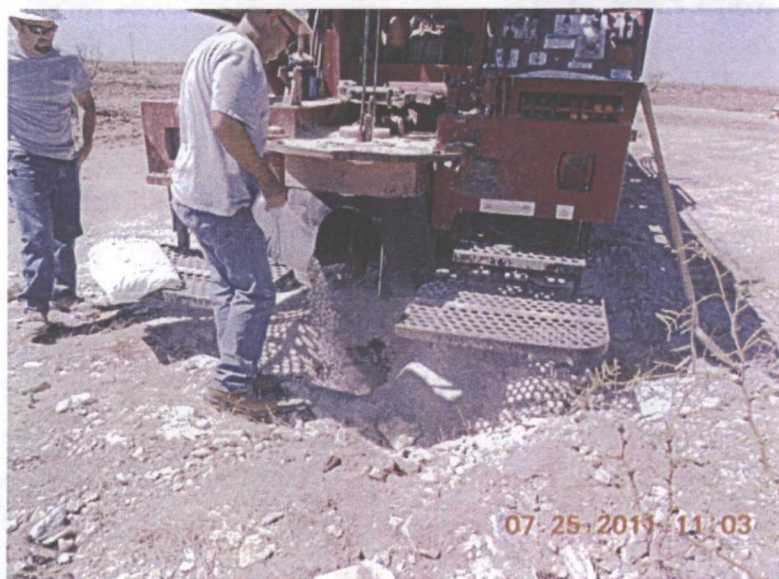
Plugging SB-1 in total with bentonite
