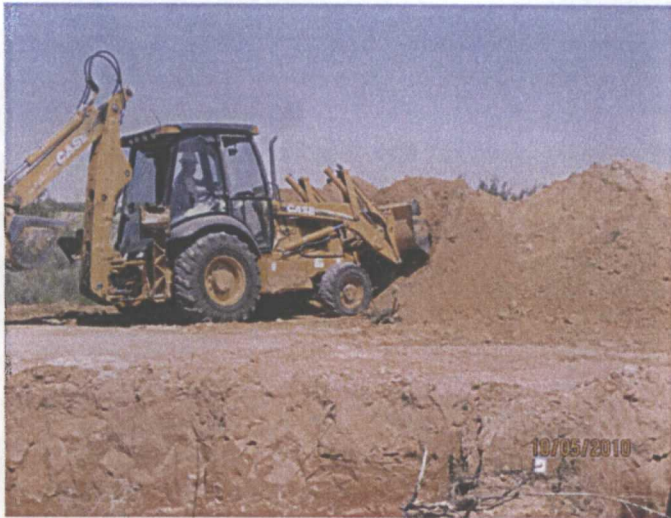
Blending backfill, facing north 10.05.10
