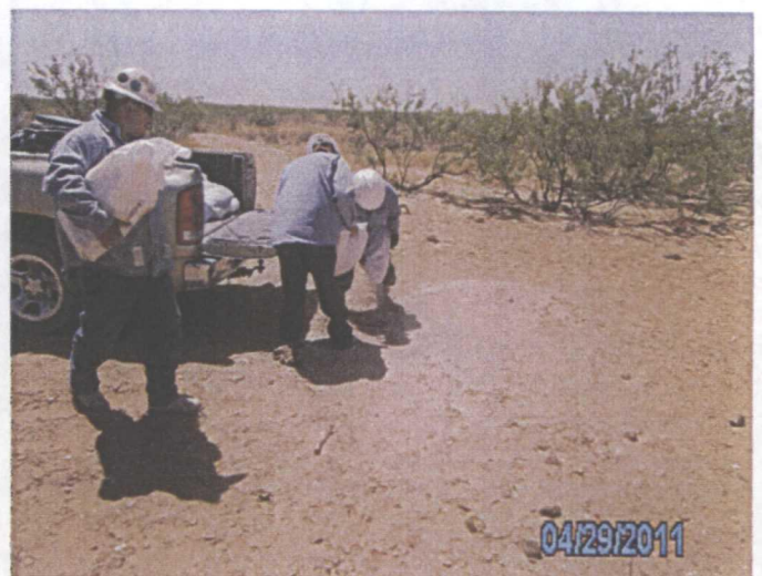
Plugging the SB in total with bentonite, facing south
