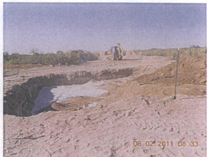
Backfilling above liner with imported soil, facing north 8/2/2011
