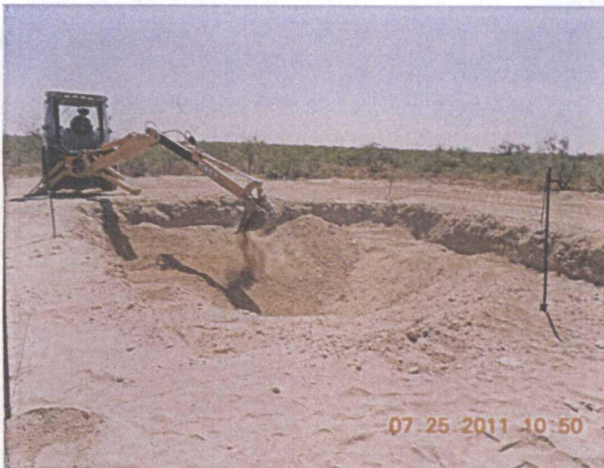
30 x 30-ft excavation being backfilled up to 4-ft BGS, facing east 7/25/2011
