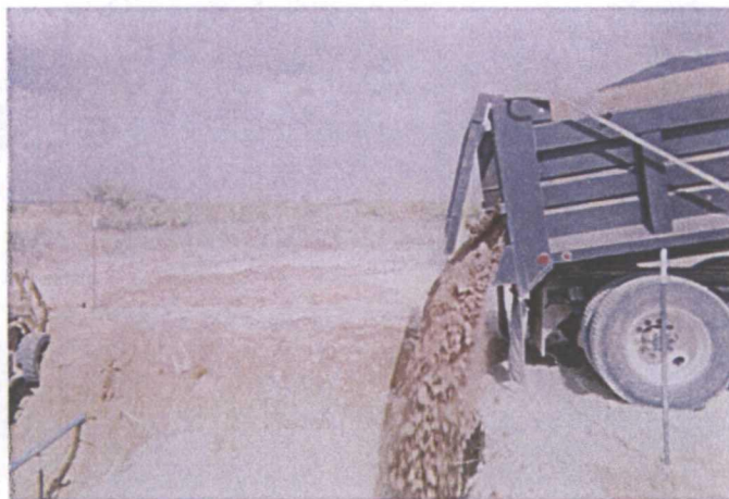
Importing clay for liner, facing north 10.21.10
