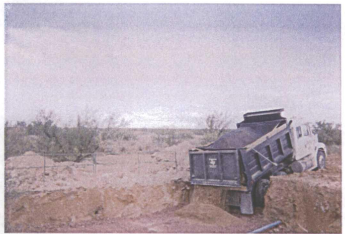
Backfilling above clay liner, facing northwest 10.22.11
