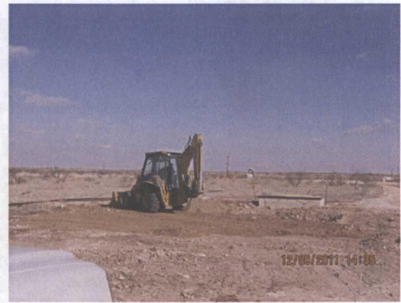
Backfilling top 6" with blow sand, facing east
