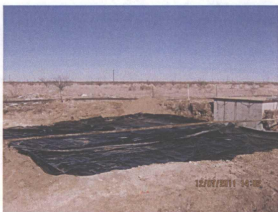
20-mil reinforced plastic liner installed at 4.5 ft BGS, facing northeast 12.7.11
