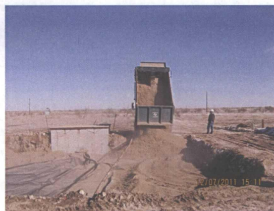
Installing 6" sand pad above liner with imported blow sand, facing east 12.7.11
