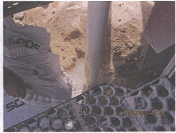
Placing the bentonite seal 10/26/11
