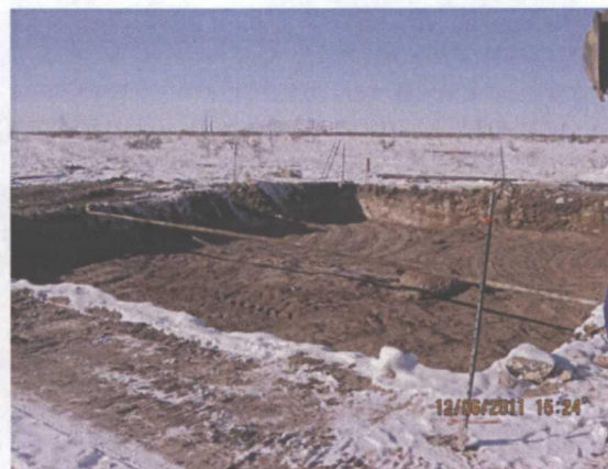
Installed bottom 6" sand pad, facing northwest 12.6.11
