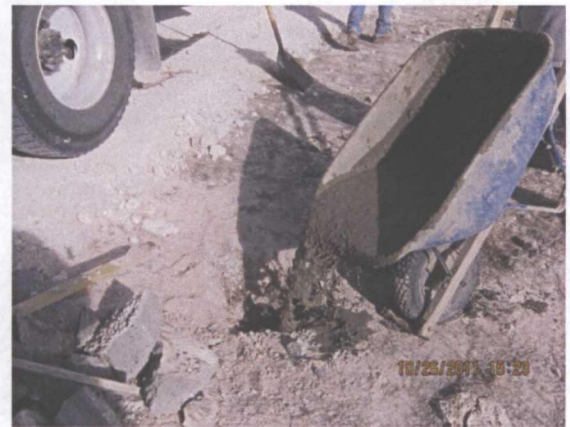
Plugging MW-1 with a 1 – 3% concrete/bentonite slurry
