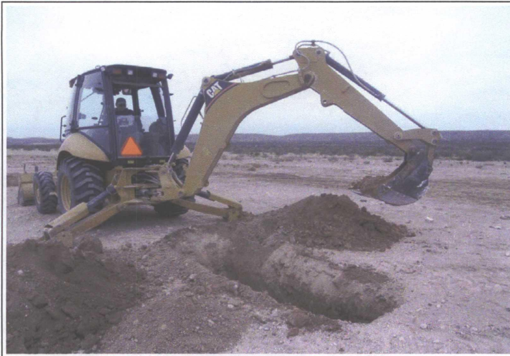
5. A total of 25 excavations to 5 ft bgs were sampled across the former Newman #1 Well site (view to the southwest).
