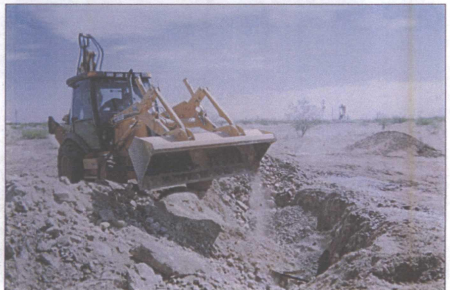
backfilling trench
