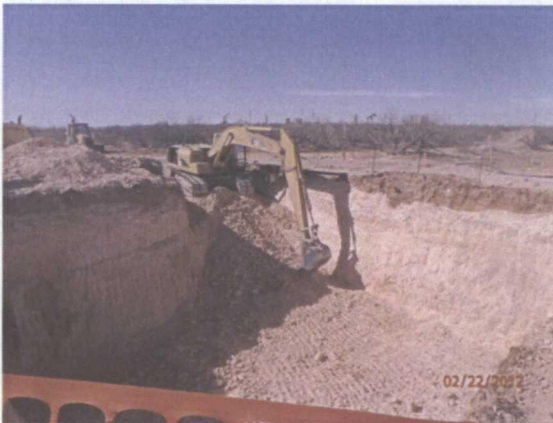
46'x51' excavation at 20' bgs, facing northwest 2/22/12
