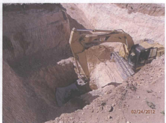
Installing sand pad above liner, facing northwest 2/24/12
