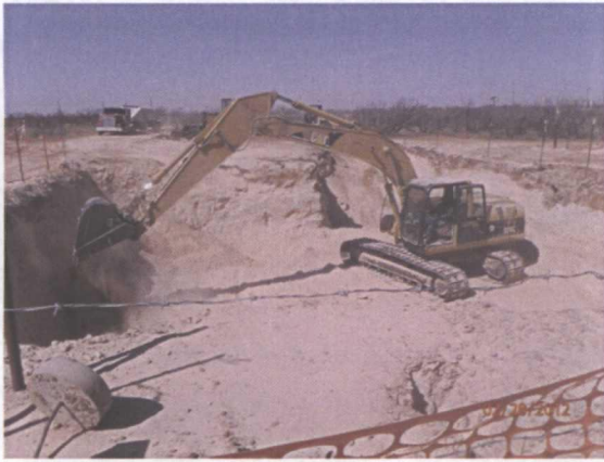
Backfilling excavation with caliche, facing south 2/28/12
