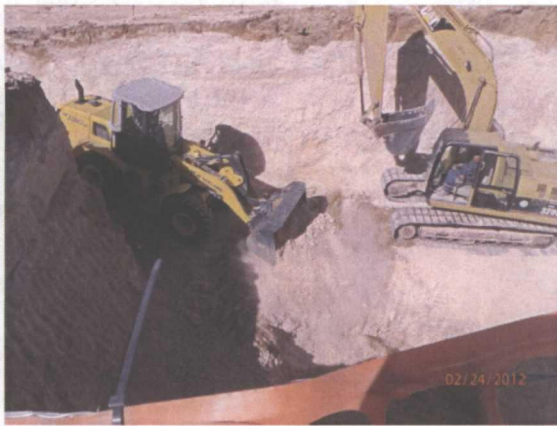
Backfilling with caliche, facing north 2/24/12
