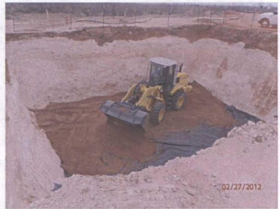
Installing 6" sand pad above liner, facing northeast 2/27/12
