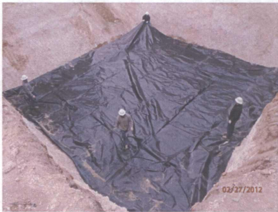
Installing the 46'x51' 20-mil reinforced liner, facing northwest 2/27/12
