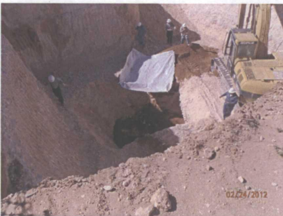
Installed liner above a 6" sand pad, facing northwest 2/24/12
