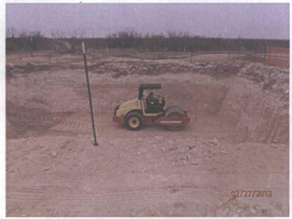
Roller packing first 3' lift, facing north 2/27/12
