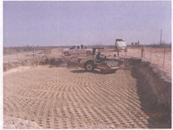
Roller packing site to 4' bgs, facing east 3/1/12
