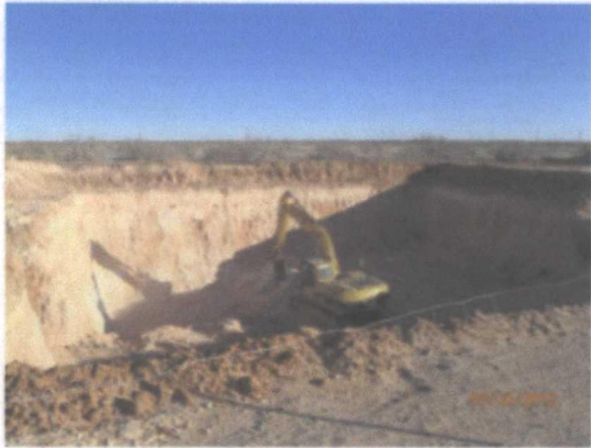
excavating the 98'x98' area to 30' bgs, facing northwest
