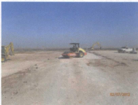
roller packing the backfilled site, facing east 2/7/2012
