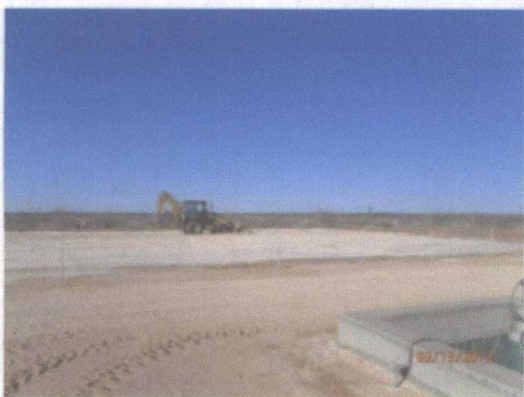
leveling the site using base coarse caliche, facing northwest 2/13/2012
