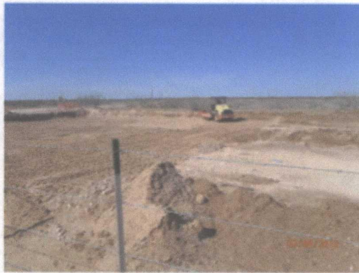
roller packing the backfilled excavation, facing northwest 2/6/2012
