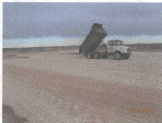
importing base coarse caliche, facing southeast 2/9/2012
