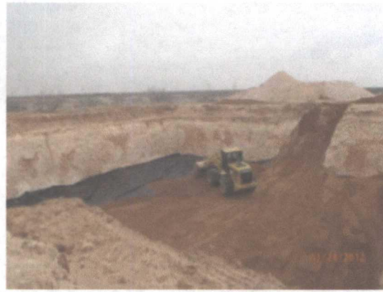
installing a 6" blow sand pad above liner, facing northeast
