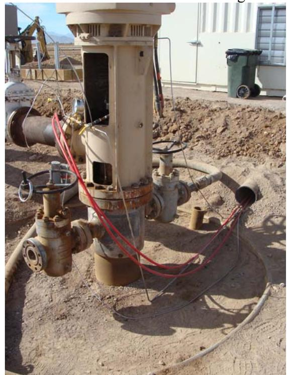
LDG 45-7 Top Mounted Water or Oil-Lubricated? Line Shaft Pump (400 HP)
