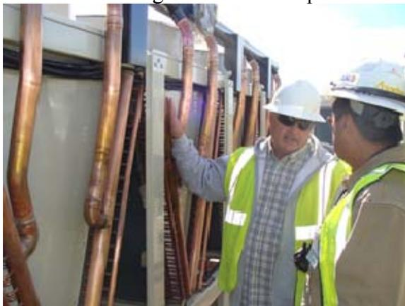
Cooling Tower Piping To Be Leak Tested
