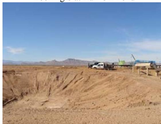
New Blowdown Pit Depression Located Near Each Production/Injection Well for Workovers, etc
