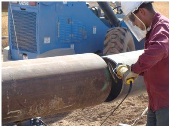
Preparing pipeline joints for welded connection
