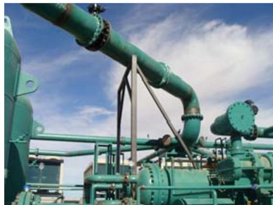
Process Lines Feed into Top of Expander Unit
