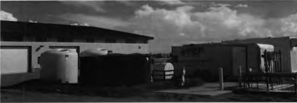
Figure 1. Produced Water Pilot Tanks, Containment, and Trailer
