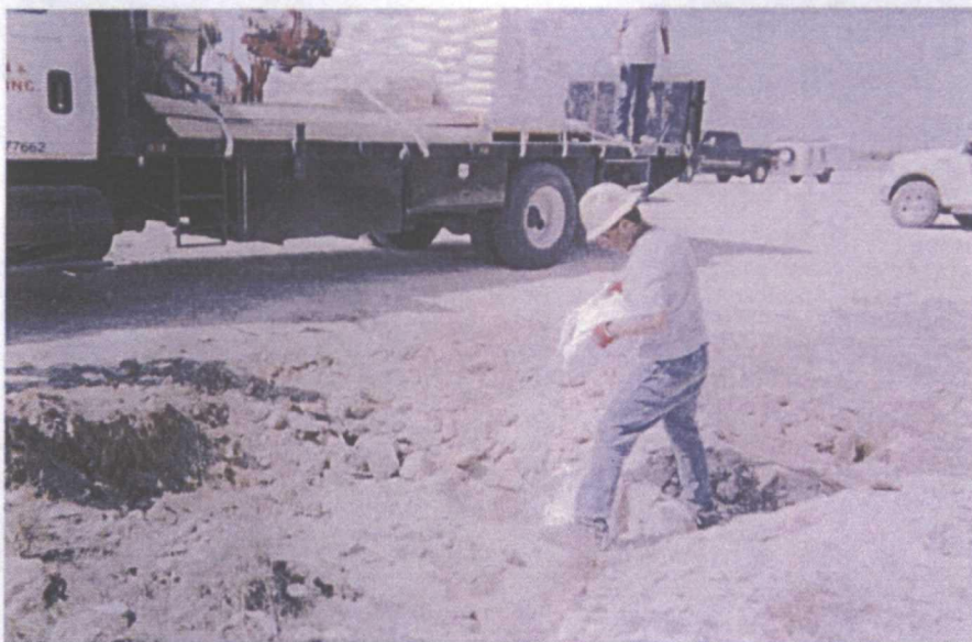
plugging SB #1 with bentonite
