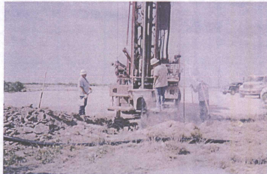
drilling SB #1 at the former junction box location
