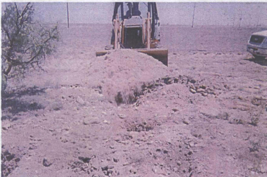
Backfilling excavation
