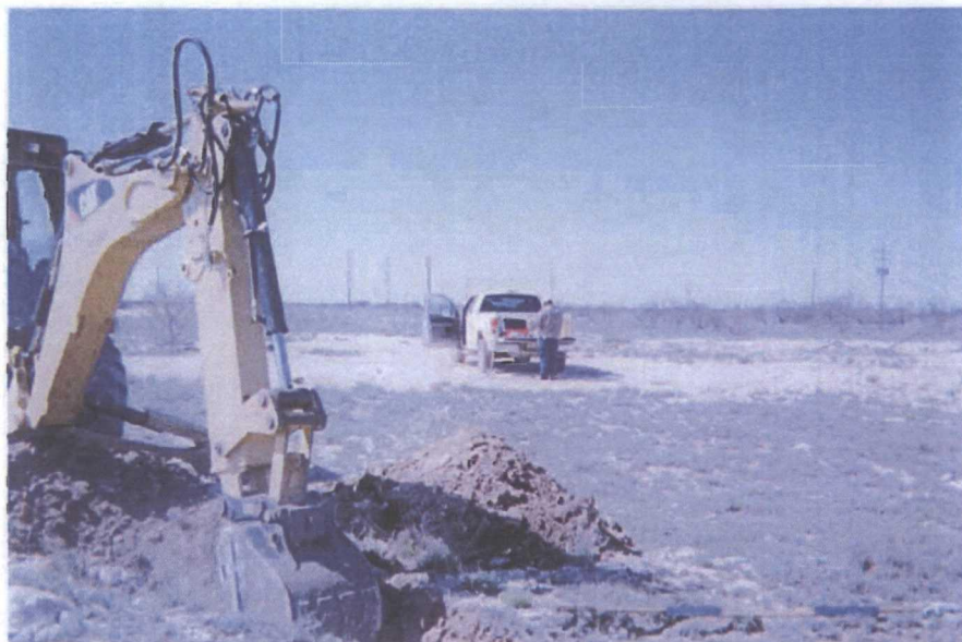
Delineation trench being excavated
