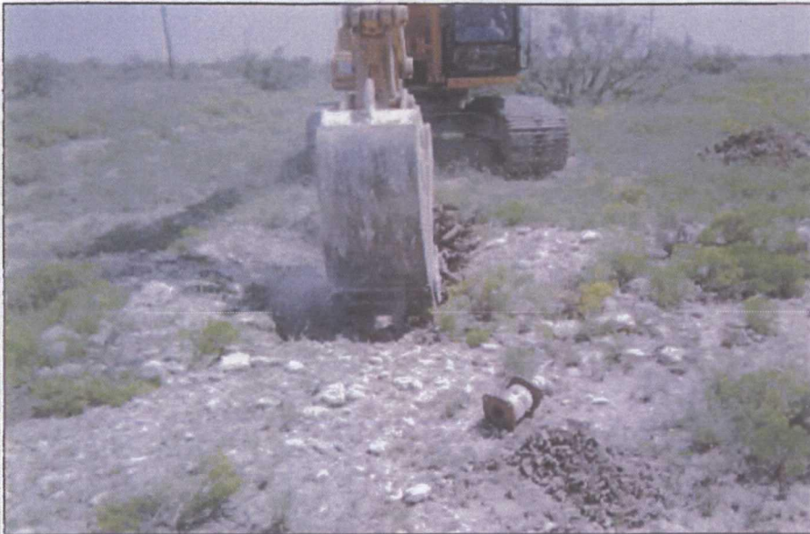
beginning junction box delineation & excavation
