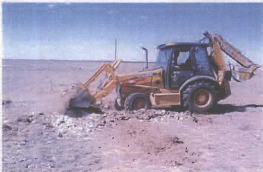
Backfilling excavation
