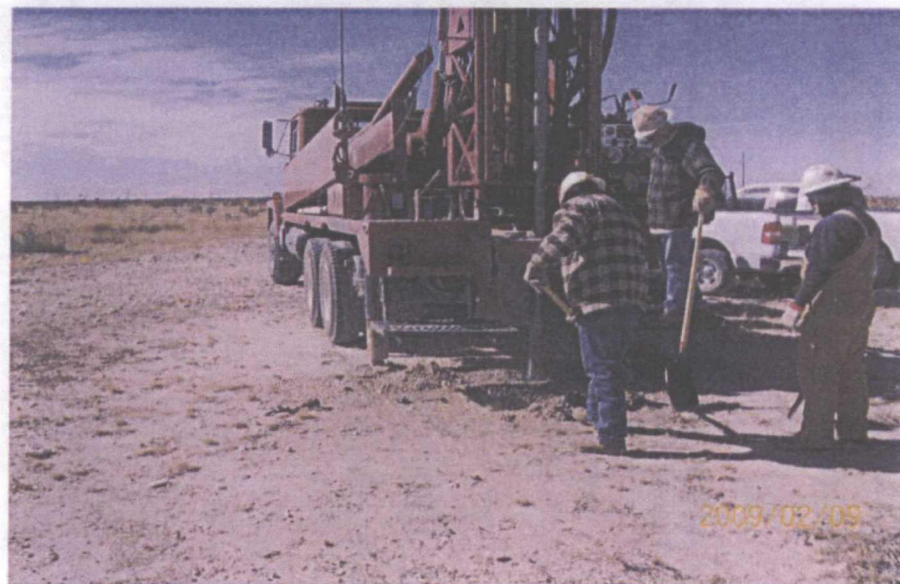
soil boring the former junction box site
