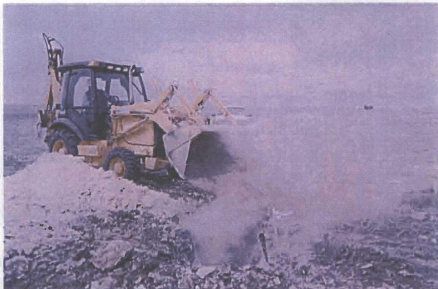
Backfilling excavation
