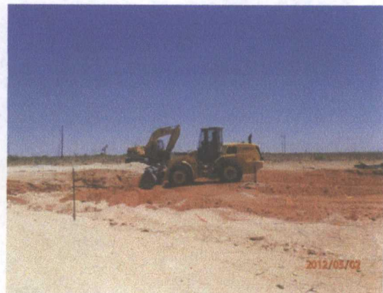
Backfilling site from 1' bgs to ground surface with sand, facing northeast 5/2/2012
