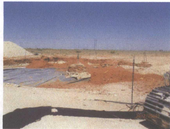
Installing 6" sand pad above liner, facing northeast 5/1/2012
