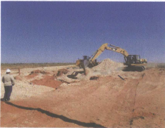
Backfilling site with caliche up to 1' bgs, facing northwest 5/2/2012
