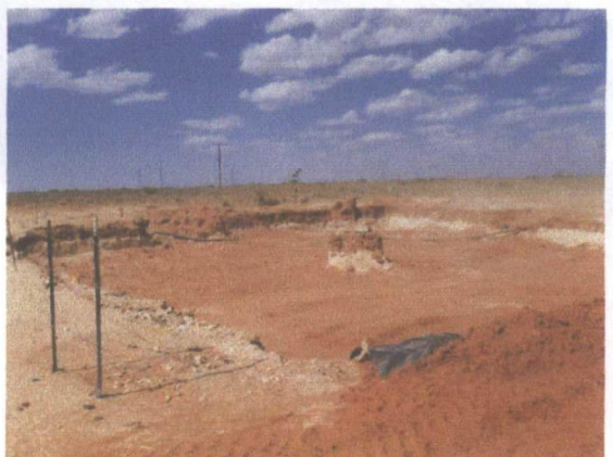
Installed bottom 6" sand pad, facing northeast 4/30/2012
