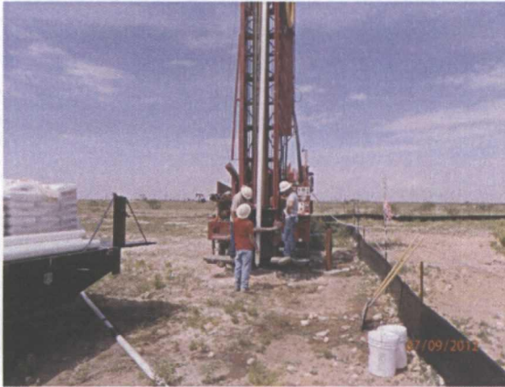
Installing the casing, facing west 7/9/12
