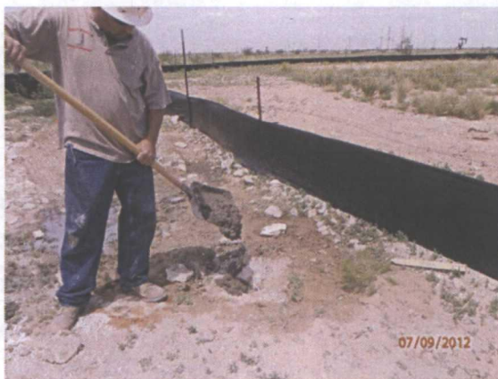
Plugging MW-1 with 1-3% bentonite/concrete slurry, facing west 7/9/12
