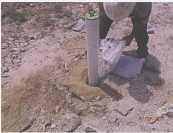
Installing the bentonite seal 7/9/12
