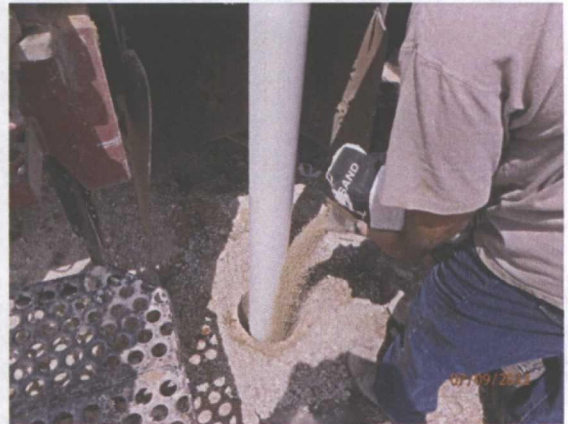
Installing the sand pack 7/9/12
