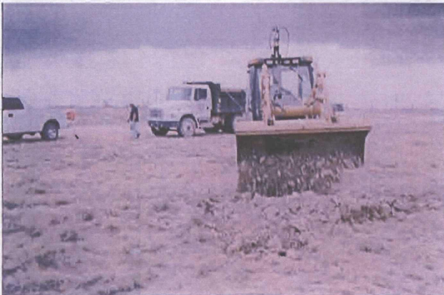
Backfilling excavation
