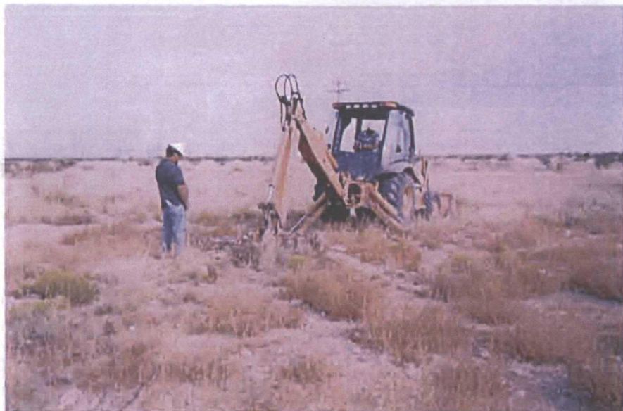
Digging initial vertical delineation trench
