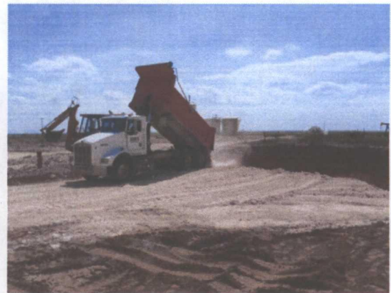
Backfilling with caliche, facing south 7/9/2012
