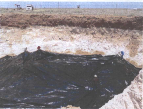
Installing 75' x 90' 20-mil reinforced liner at 25' bgs, facing west 7/2/2012
