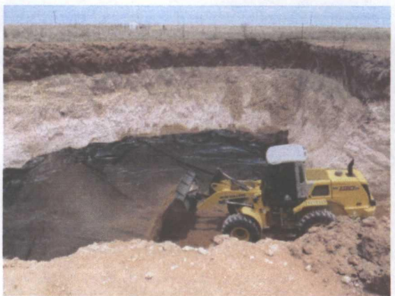
Installing 6" sand pad above liner, facing north 7/2/2012
