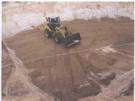
Installing 6" bottom sand pad, facing west 7/2/2012
