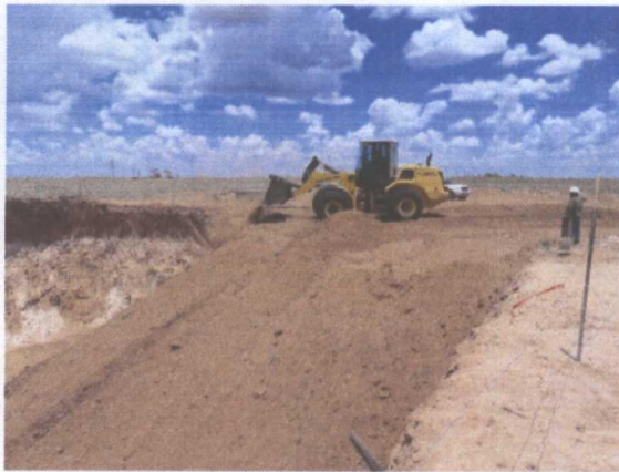
Backfilling with imported topsoil, facing east 7/5/2012
