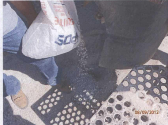
Plugging SB-7 in total with bentonite 8/9/12
