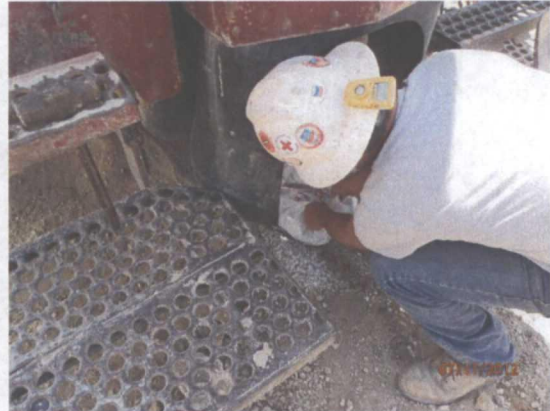
Plugging SB-2 in total with bentonite
