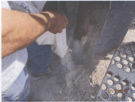
Plugging SB-6 in total with bentonite
