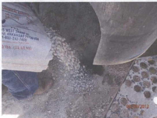
Plugging SB-8 in total with bentonite 8/9/12
