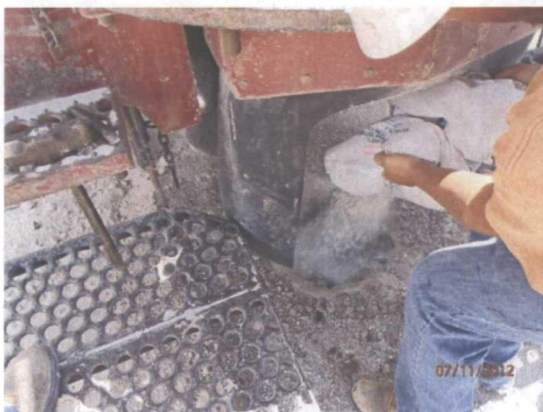
Plugging SB-3 in total with bentonite
