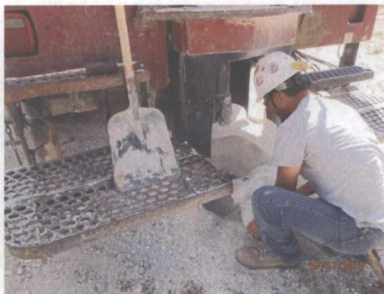
Plugging SB-4 in total with bentonite
