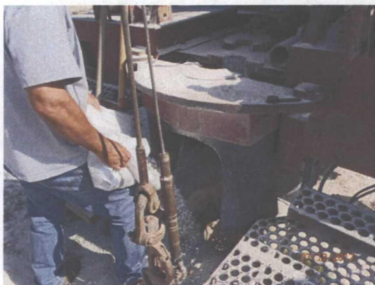
Plugging SB-5 in total with bentonite
