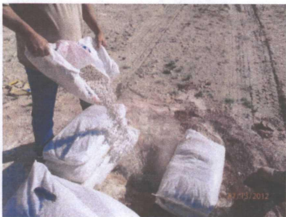
Plugging SB-2 in total with bentonite 7/13/12
