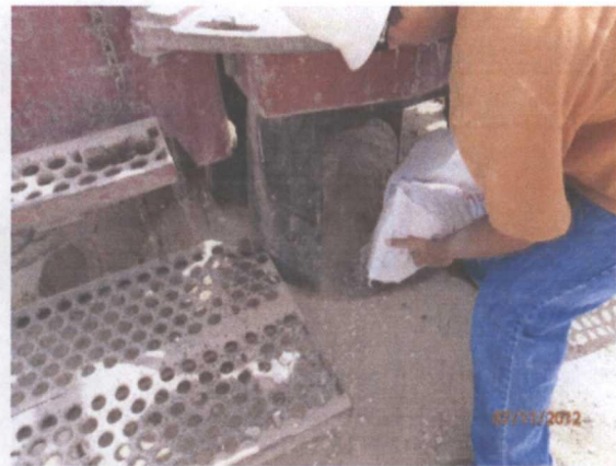
Plugging SB-1 in total with bentonite
