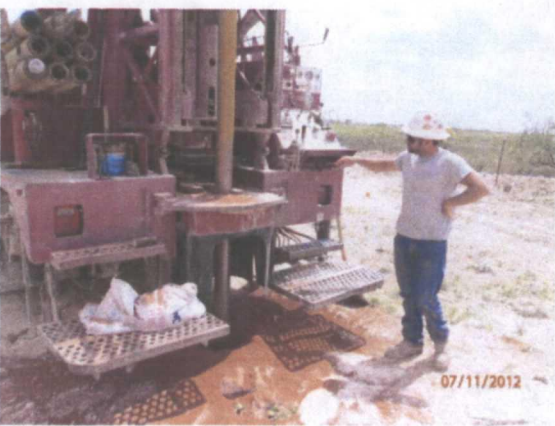
Drilling into red bed clay at SB-2
