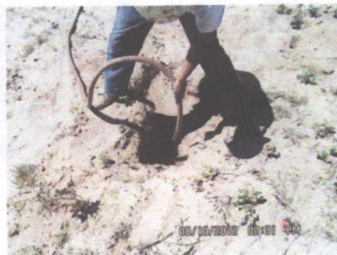
Each MW was filled with Cement Type I-II and 1-3% bentonite grout.
