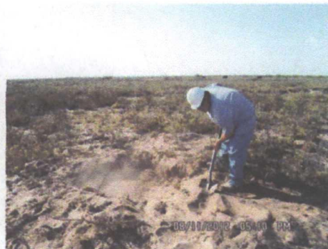
24 hours later-each hole was backfilled with native soil.
