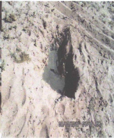
Holes filled with cement grout
