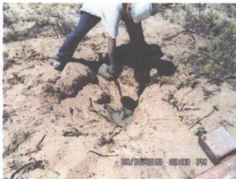
Topping of each hole to counter slumping.
