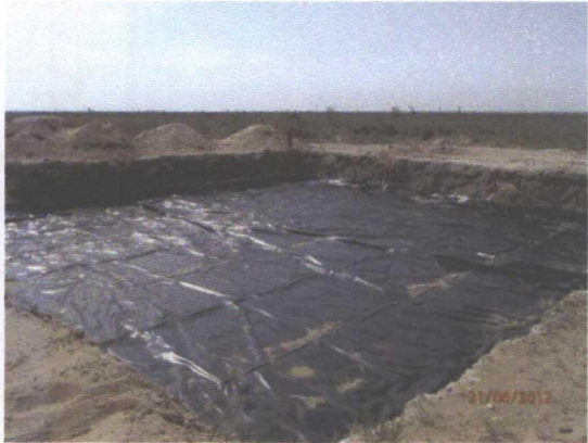
Liner installed, facing southeast 6/21/2012
