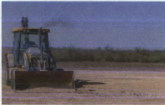
Figure 2: Backfilling a "Y" shaped trench with caliche.
