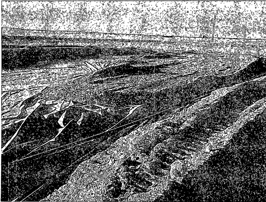
Pad area - 1.0' of caliche material top of liner
