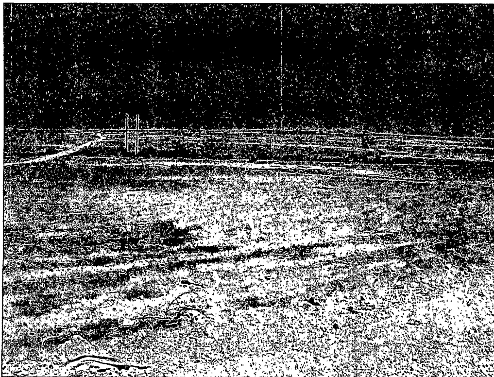
Reserve pit and north area - backfilled with 2.0 to 3.0' of clean topsoil
