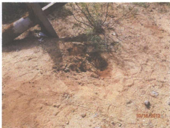
Completed plug and abandonment of MW-2, facing south 10/16/12
