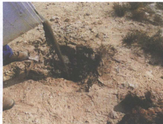
Plugging MW-5 with a 1-3% bentonite/concrete slurry and a 3 ft concrete cap
