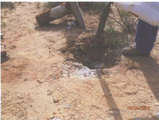
Plugging MW-2 with a 1-3% bentonite/concrete slurry and a 3 ft concrete cap 10/16/12
