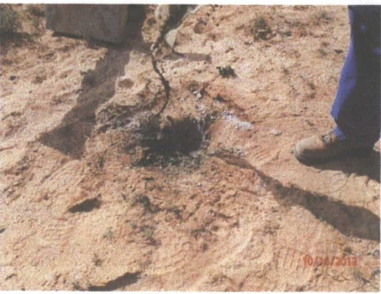
Plugging MW-4 with a 1-3% bentonite/concrete slurry and a 3 ft concrete cap 10/16/12
