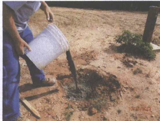
Plugging MW-1 with a 1-3% bentonite/concrete slurry and a 3 ft concrete cap 10/16/12
