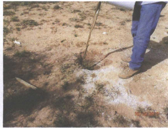
Plugging MW-3 with a 1-3% bentonite/concrete slurry and a 3 ft concrete cap 10/16/12
