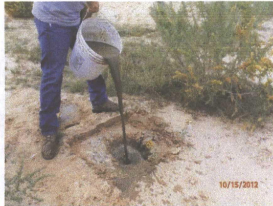
Plugging MW-1 with a 1-3% bentonite/concrete slurry with a 3 ft concrete cap 10/15/12
