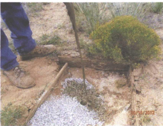
Plugging MW-2 with a 1-3% bentonite/concrete slurry with a 3 ft concrete cap 10/15/12
