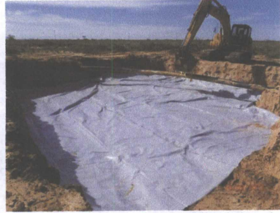
excavation complete, with a 20-mil, reinforced liner installed, facing southwest 10/9/2012
