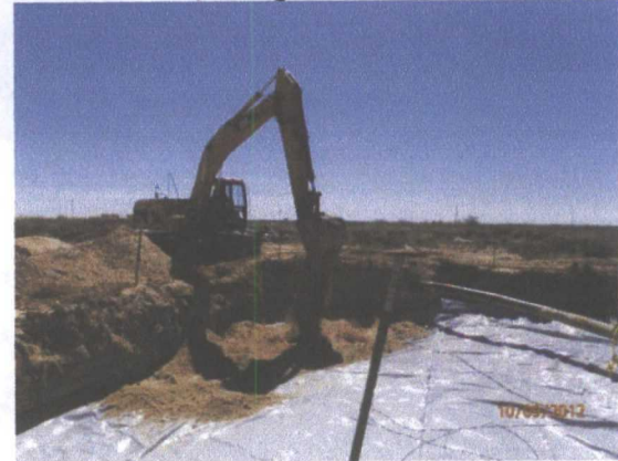
backfilling the excavation with blow sand, facing south 10/9/2012
