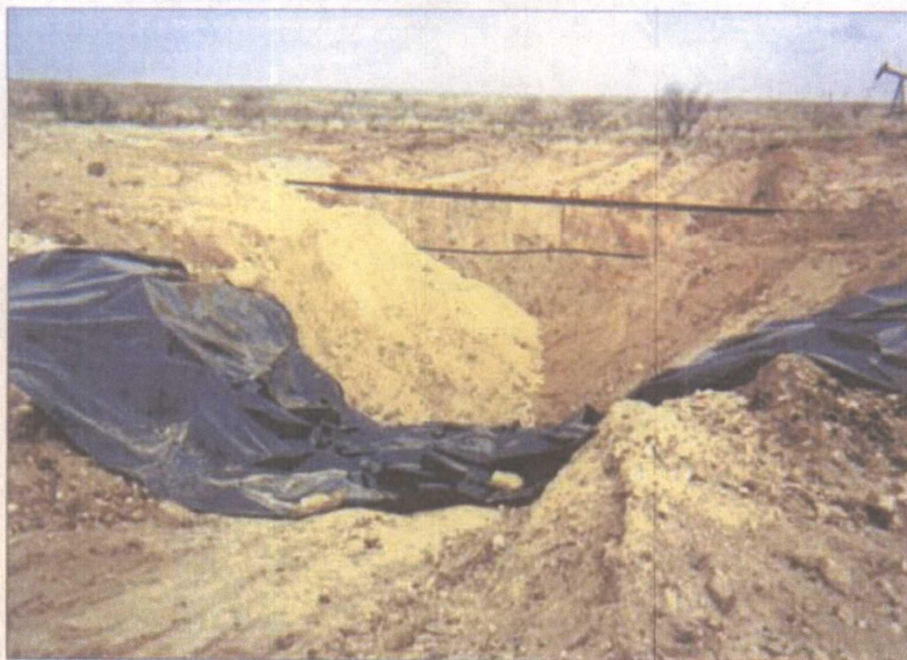
Backfilling Poly Liner
