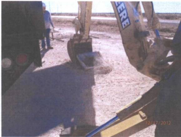
Pulling concrete base free of PZ-4, facing southwest 12/17/12
