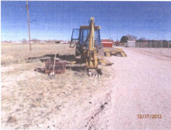
Pulling concrete base free of BS-3, facing east 12/17/12
