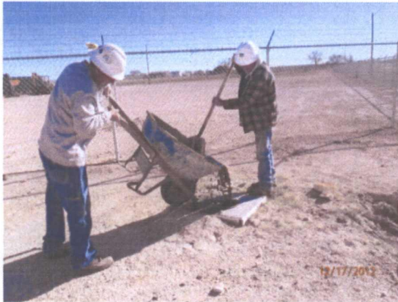
Plugging MW-3R with a 1-3% bentonite/concrete slurry with a 3 ft concrete cap, facing south 12/17/12
