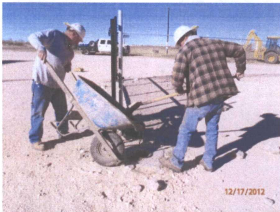
Plugging PZ-3 with a 1-3% bentonite/concrete slurry with a 3 ft concrete cap, facing north 12/17/12
