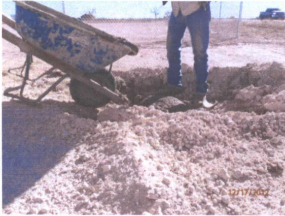
Plugging MW-3 with a 1-3% bentonite/concrete slurry with a 3 ft concrete cap, facing south 12/17/12
