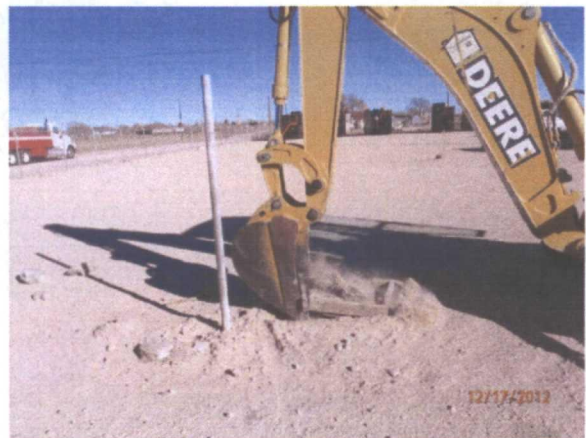
Pulling concrete base free of PZ-3, facing east 12/17/12
