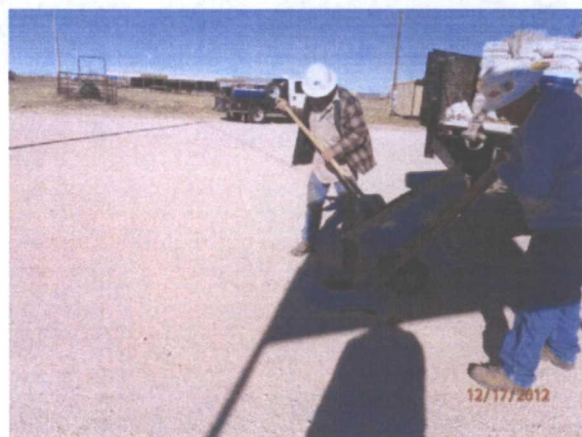
Plugging PZ-4 with a 1-3% bentonite/concrete slurry with a 3 ft concrete cap, facing north 12/17/12
