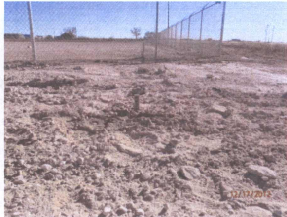
MW-3 plugged and abandoned, facing south 12/17/12
