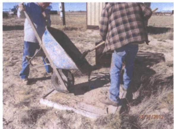
Plugging BS-3 with a 1-3% bentonite/concrete slurry with a 3 ft concrete cap, facing north 12/17/12
