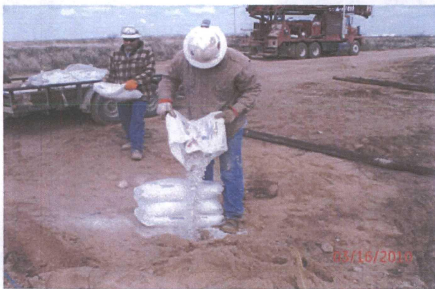
Plugging soil bore # 1 with bentonite
