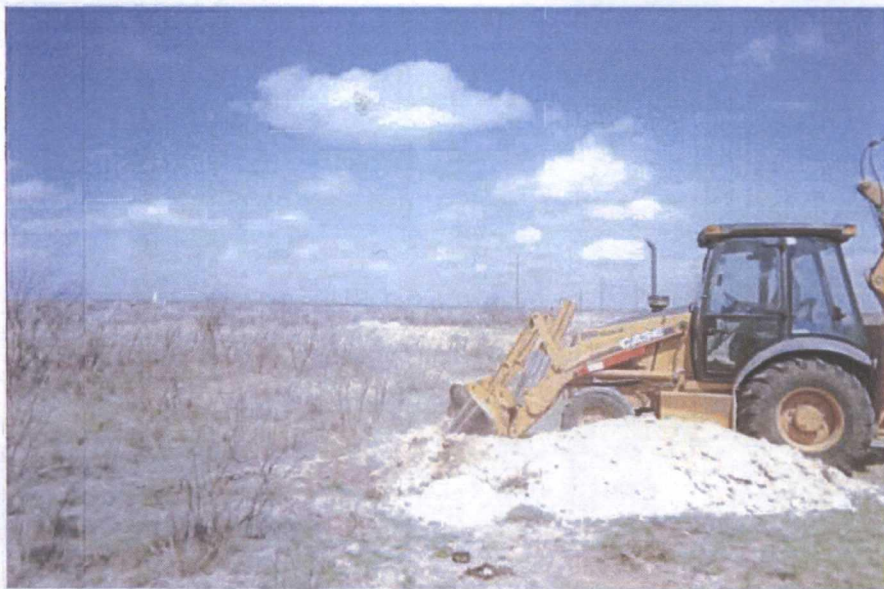
Backfilling excavation
