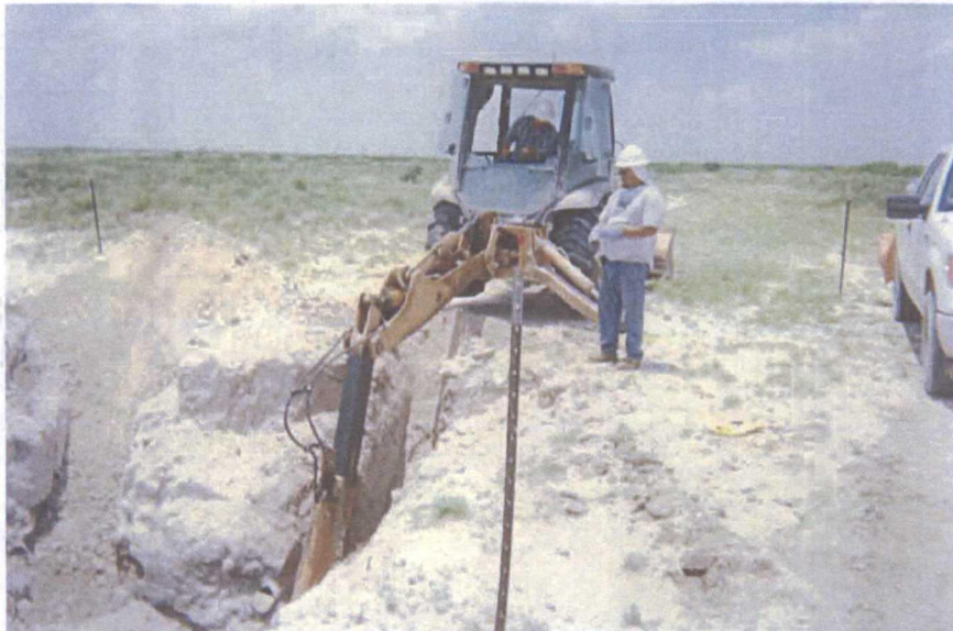
Delineation trench being excavated
