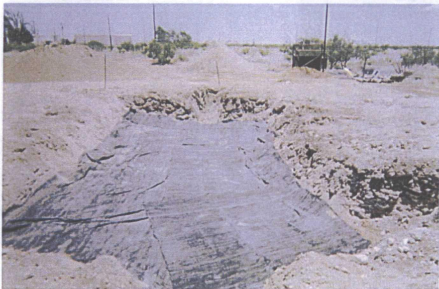
45X20 geosynthetic liner installed
