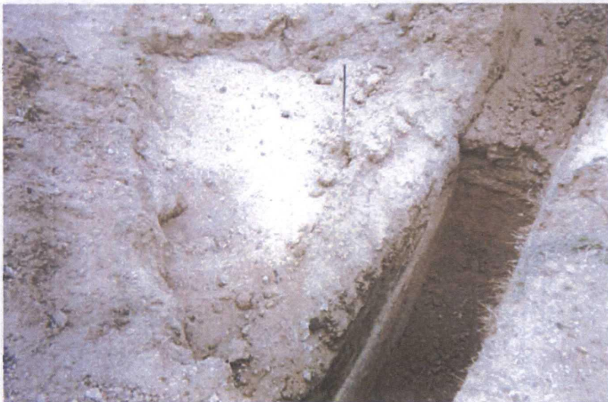
Final excavation 5x3x7 4/13/2010
