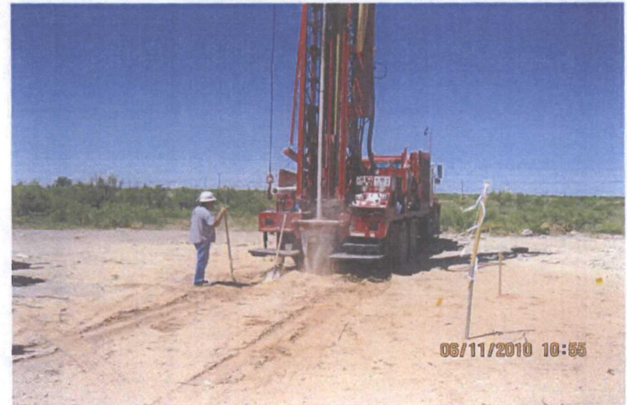
Drilling soil bore
