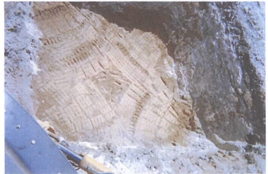
6" blow sand pad above plastic liner
