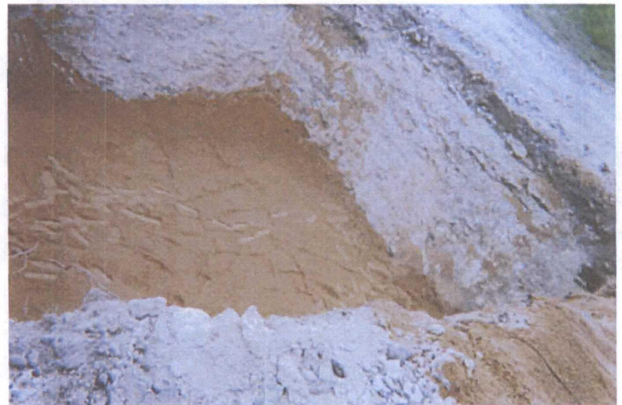
6" blow sand pad below plastic liner
