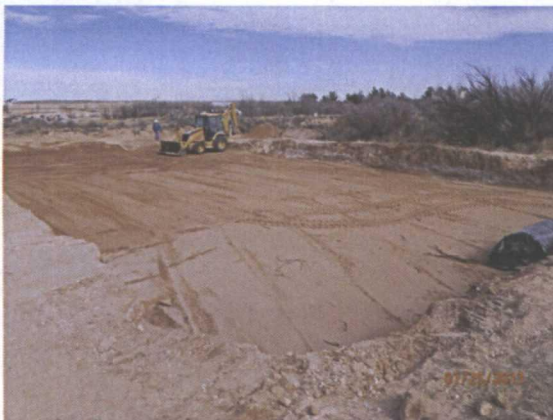
Installing sand pad below liner, facing northeast 1/25/13
