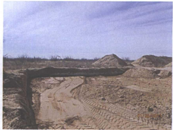
Padding above liner completed, facing southwest 1/28/13
