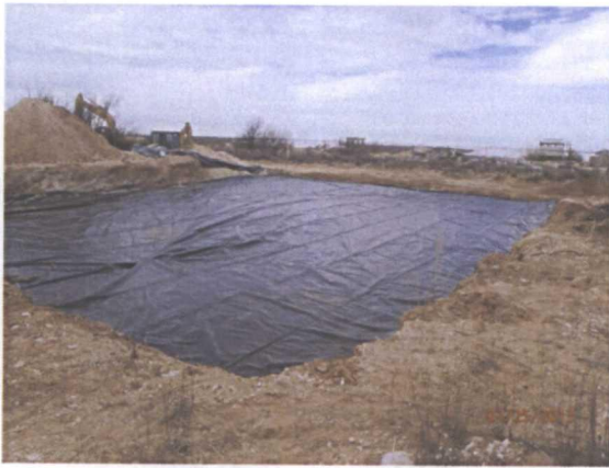
Liner installation completed, facing northwest 1/25/13
