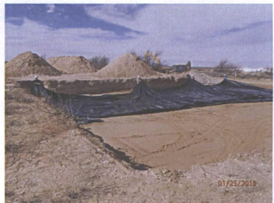
Installing liner, facing northwest 1/25/13
