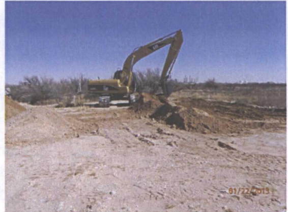
Scraping caliche to 1'6", facing west 1/22/13
