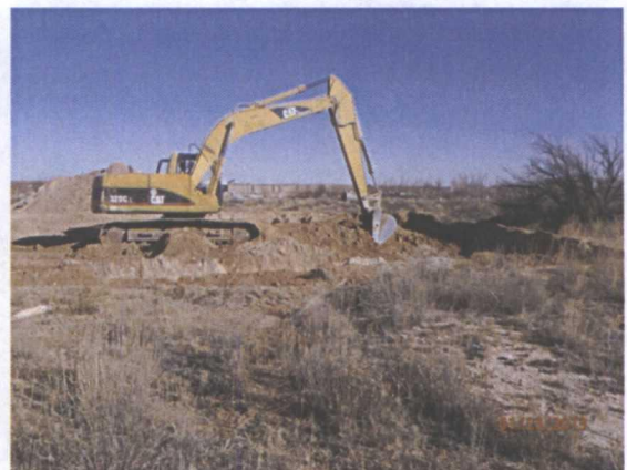
Excavating the site down 4'6", facing north 1/23/13
