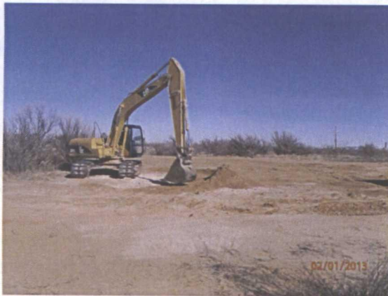
Spreading top soil over site, facing east 2/1/13
