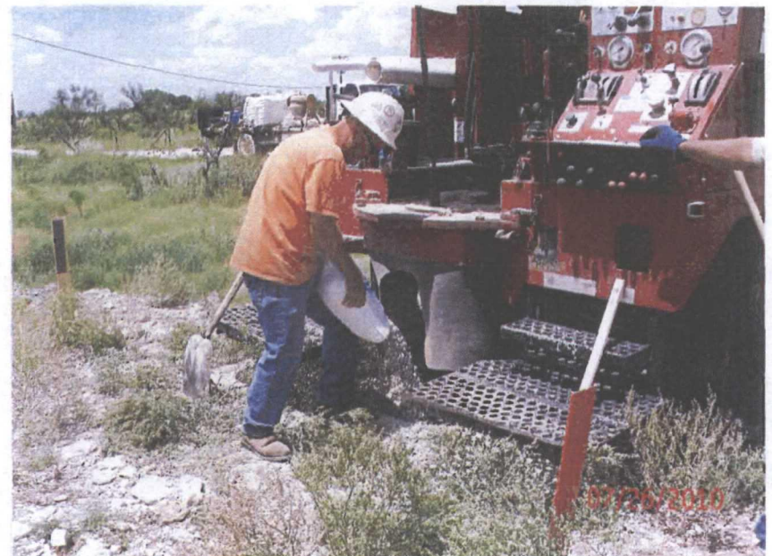
Soil Bore plugged with bentonite
