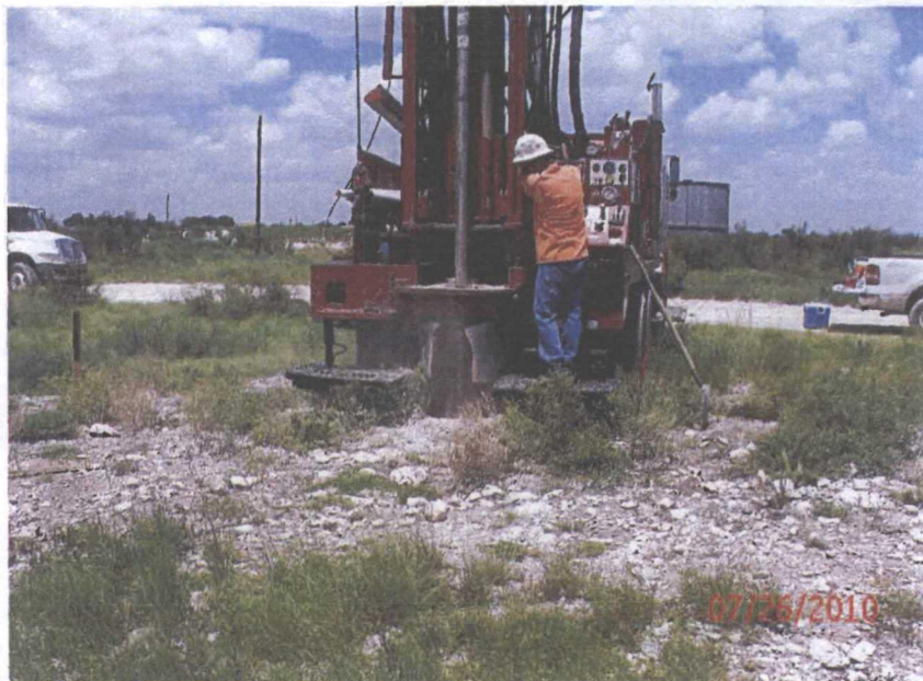
Drilling Soil bore
