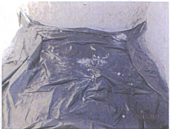
Installed 30'x30' liner @ 12' bgs
