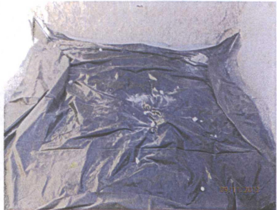
Installed 30'x30' liner @ 12' bgs
