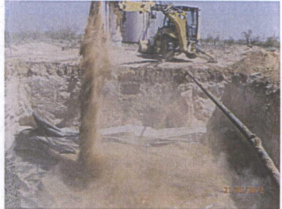
Installing 6' sand pad above liner, facing east
