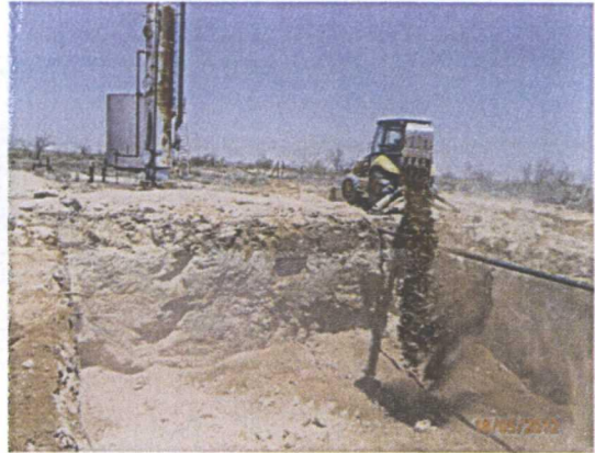
Installing 6' sand pad below liner, facing north
