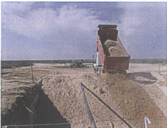
Backfilling with imported soil facing south
