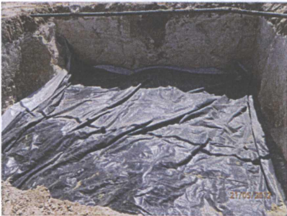
Installed 25'x20' liner @ 12' bgs, facing west
