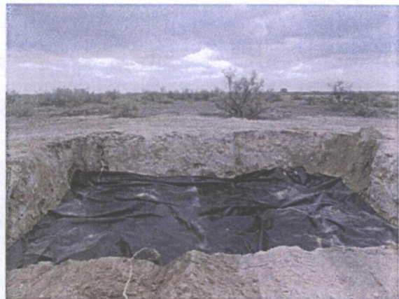
Installing 30'x30' 20 mil plastic liner @ 6' bgs 10/12/2012
