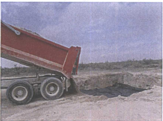
Backfilling with imported soil 10/12/2012
