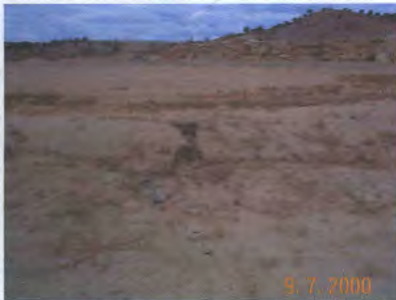
Erosion across the last terms southeast corner. Reconstruction needed
