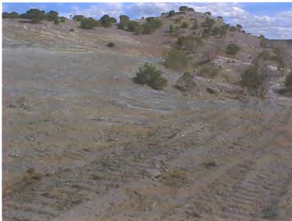
Secondary hillside diversion guides storm water to gabion structure
