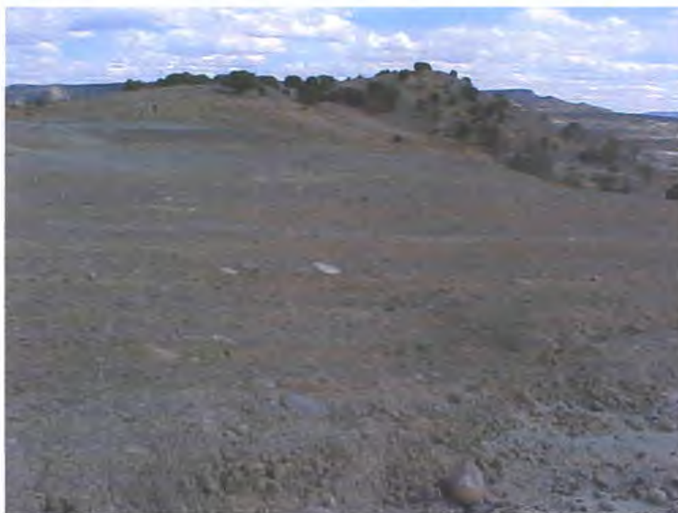
Primary diversion along left center of photo guides storm water to gabion through broad channel at small cedar (upper right center)
