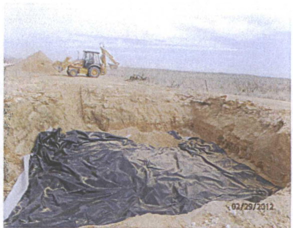
Installing liner, facing east
