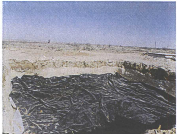
Installing 30'x30' liner @ 6' bgs, facing west
